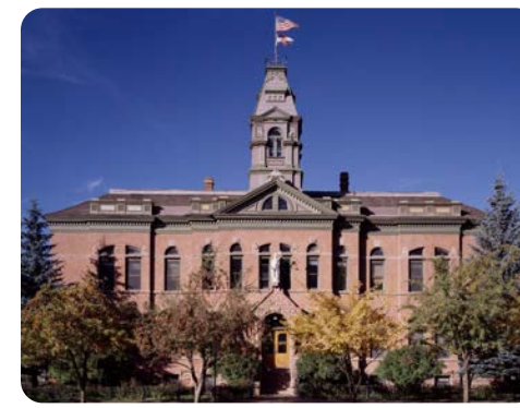
Pitkin County Courthouse
